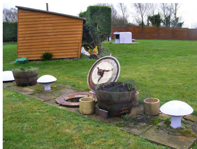
The surface features of the BX shelter at Pluckley. The Pluckly ROC Post is seen in the background.
